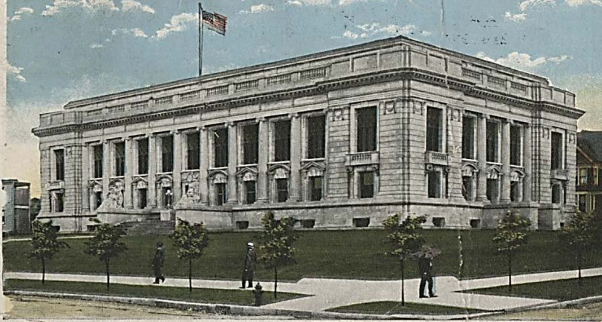
Supreme Court Building, Springfield, Ill.
